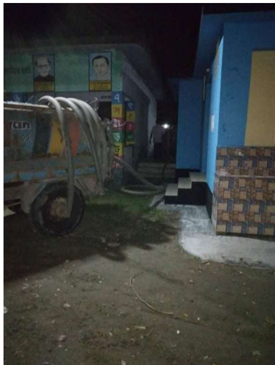
(b) Cleaning of septic tank by using automatic vaccu-truck at Gaibandha
